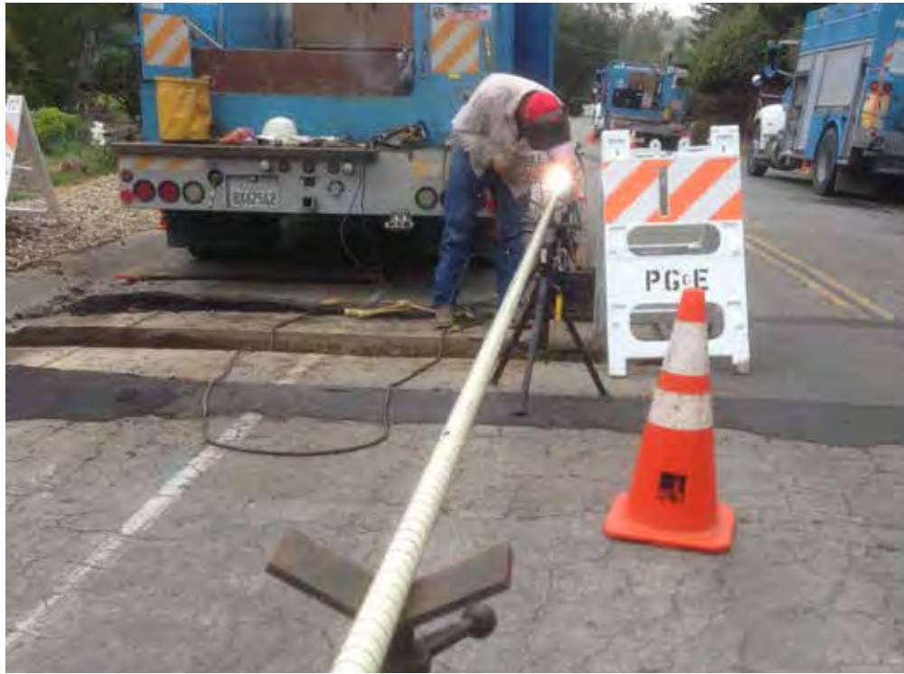
A PG&E welder cuts a new steel lateral for installation.
